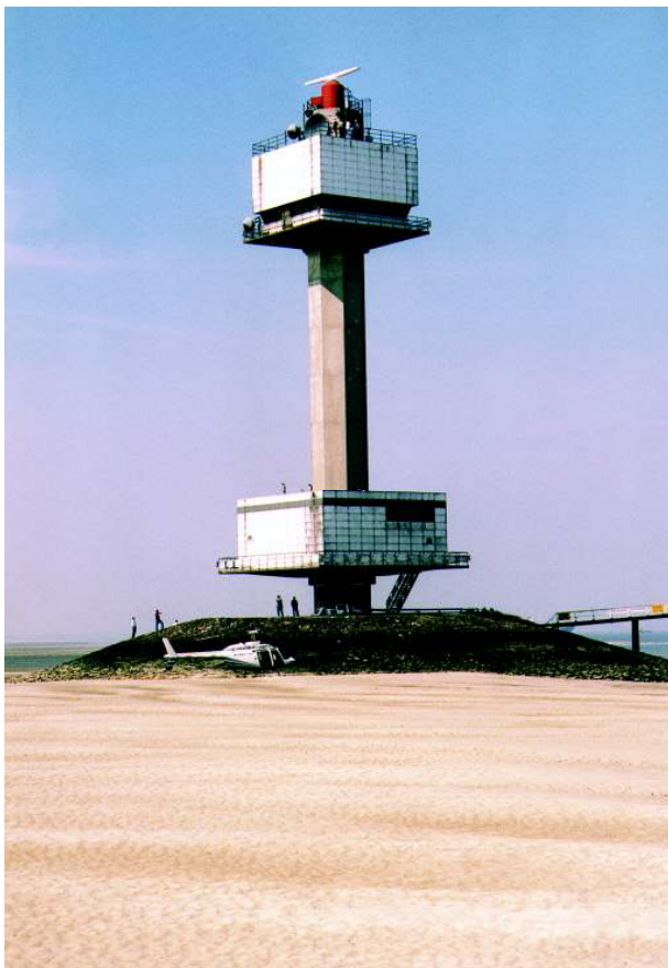
Radar is a key requirement for most VTS. Siting the antenna in the right location and obtaining adequate height requires much consideration. Some solutions: above, an automatic facility at Oostdyckbank, ten miles off the Belgian coast (Flemish Waterways); below left, at Saeftinghe, and below right, the old tower a La Maddalena, Italy. (Italian Coast Guard)
