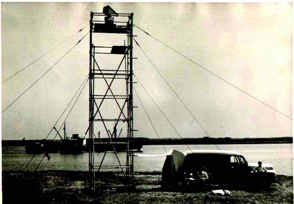
Fig. 1.1: VTS test site Rotterdam 1948 Source: Photo, collection D. Zwijnenburg.
